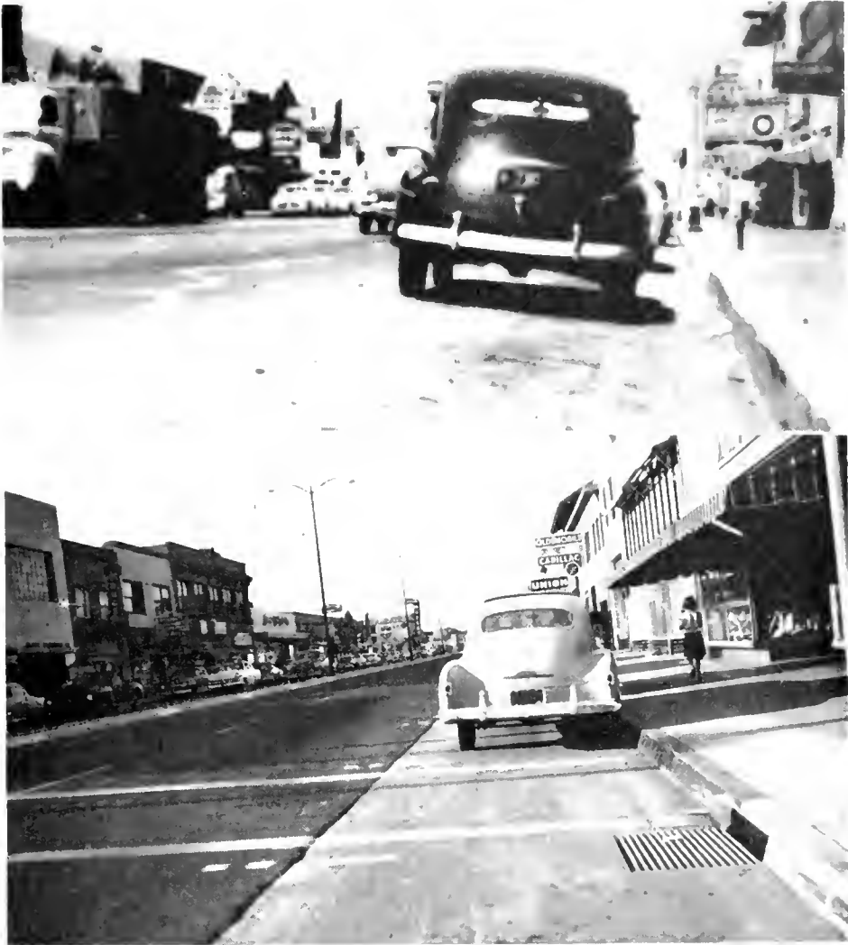
UPPER—Photo taken in 1951. LOWER—Photo taken in 1955. Both on Monterey Street showing the difference in typical parking conditions. The high crown and high curb shown in the earlier photo made it difficult to open car doors unless the car was parked same distance from curb, as shown in the photograph.
